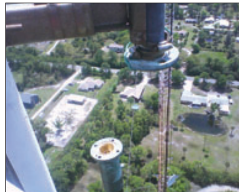
Mid - Air Repairs!
