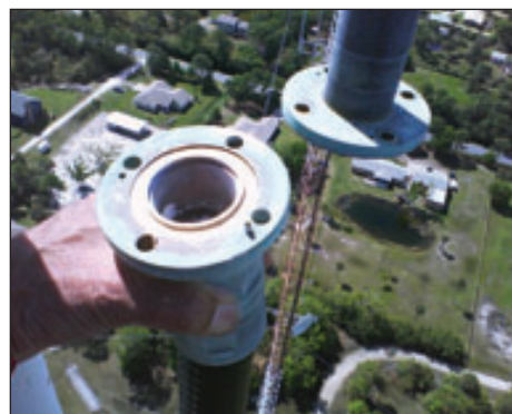
Antenna being lowered to connect the transmission line.
